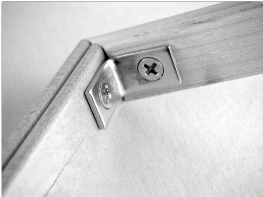
FIGURE 9-5: Detail of an inner frame corner brace
