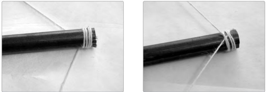
FIGURE 23-9: Detail of the string wrapping at the end of a spar (back side at left; sail side at right)
