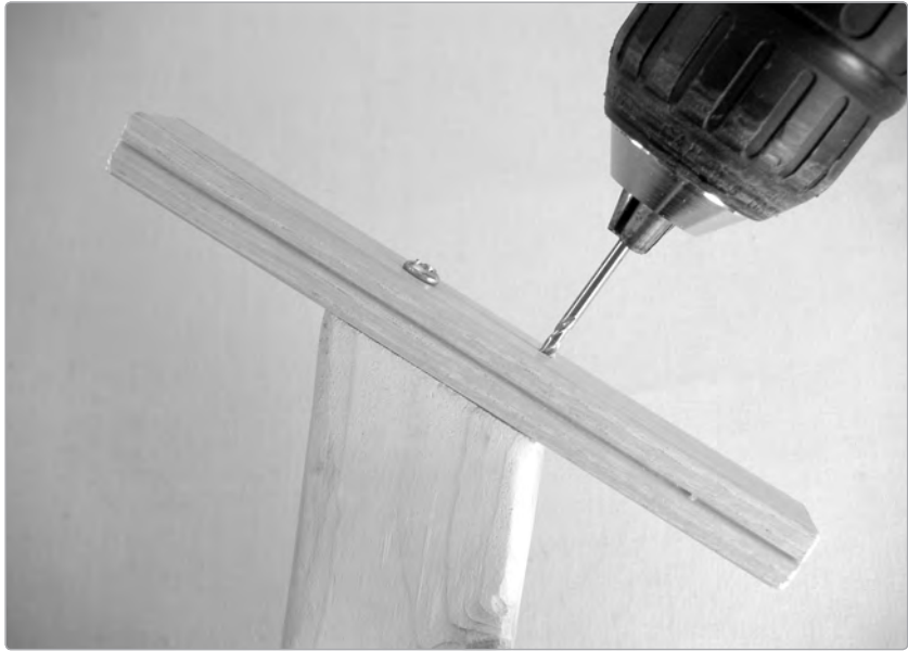
FIGURE 24-6: Drilling a guide hole in the grip
