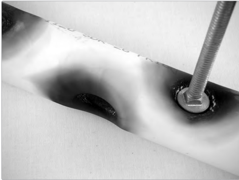
FIGURE 11-7: Adding a new dimple; note the completed dimples to the left
